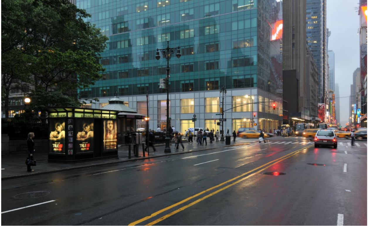
View of 1095 Avenue of the Americas from 42 nd Street.
